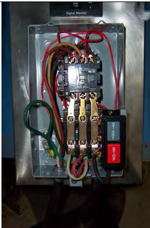
Figure 2.3.1 CB-260 Control Box inside view
