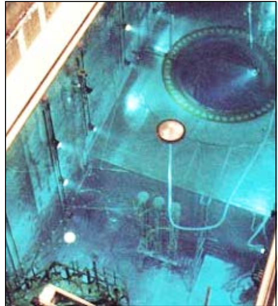
SK-175 Skimmer in operation at a PWR
